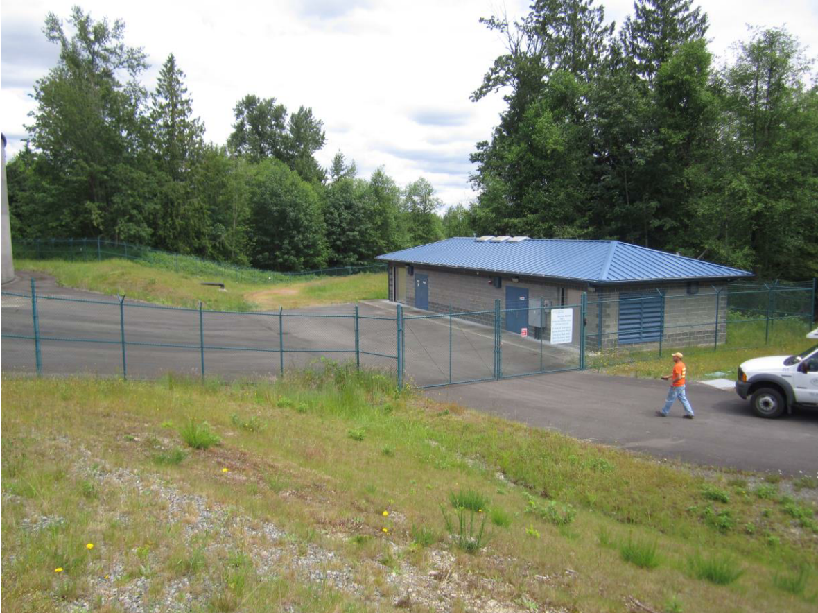
Peaking Storage Booster Pump Station
